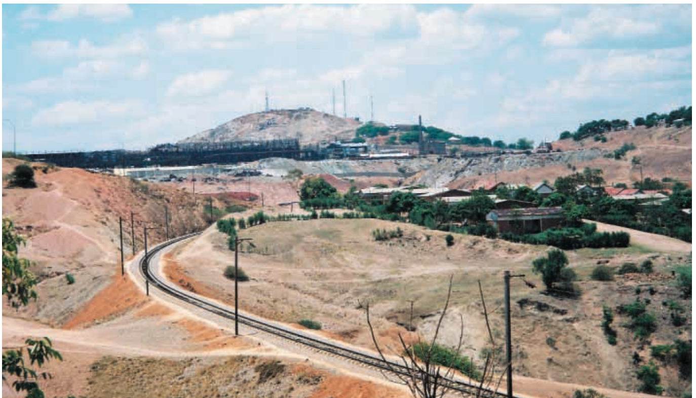
Railway line used to transport copper and cobalt between Likasi and Lubumbashi, Katanga, November 2005.
